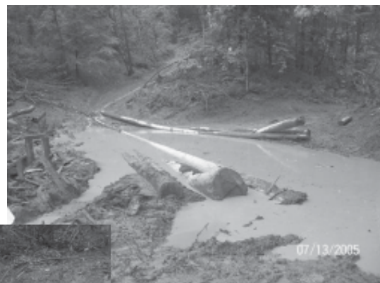
Above: Skid trail running downhill into flat next to stream. Notice flow of muddy water coming down skid trail from uphill seep. Water bar or other water control was needed to divert this flow before it gets to the bottom next to the stream.
