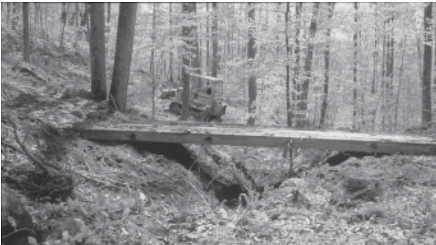
**Bridge Panels should extend 4-6 feet on each side of the stream bank for support.**
